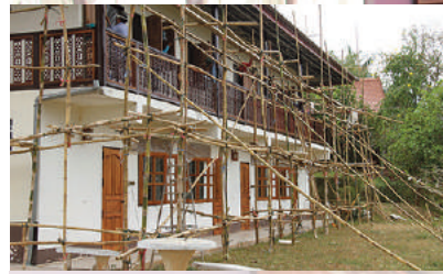
Guest rooms and storage rooms
