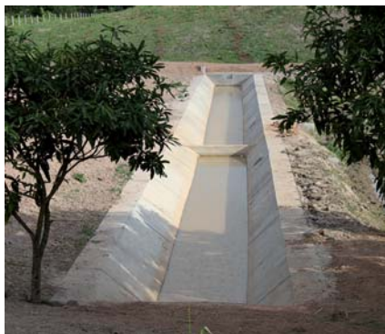
Improvement of the irrigation system
